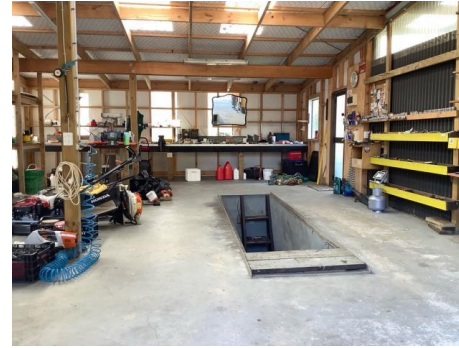
Service pit in shed
