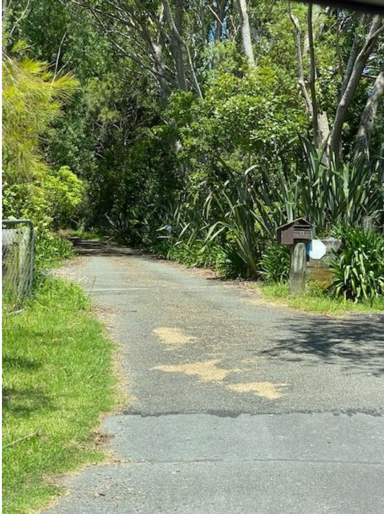
Figure 7: Photograph of entrance to existing access to be upgraded (Lot 5 DP 53393)
