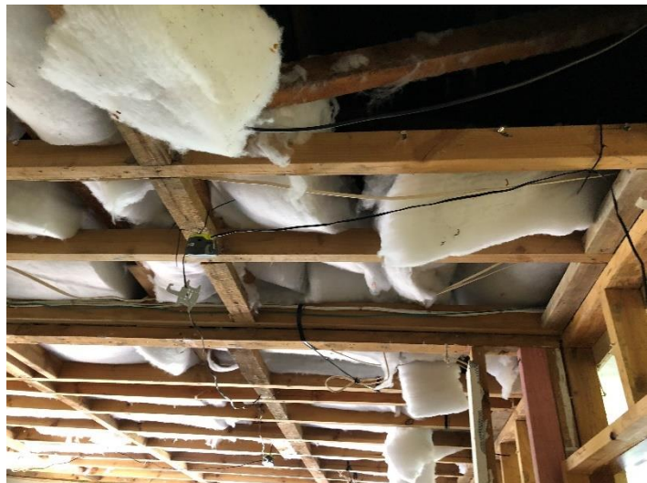
Fig 2: Ceiling over corridor
