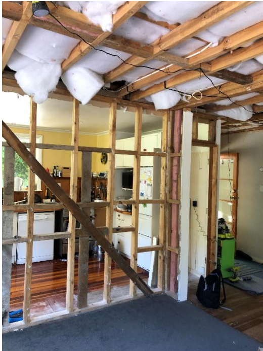
Fig 1: Wall to be removed
