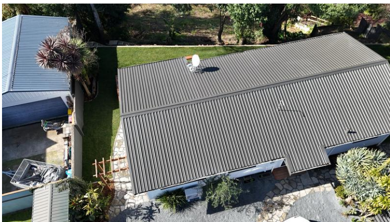
Photo 3 Profiled metal gable roof construction with nail fixings.
